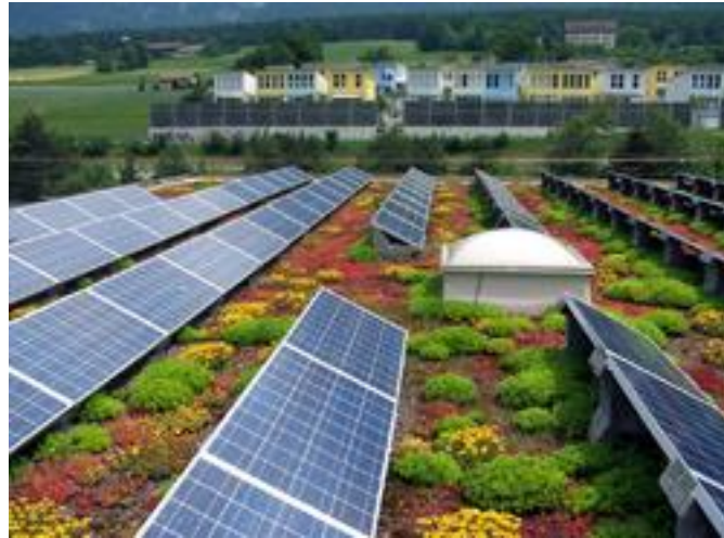
Figure 14.2. Solar PV installed on a green roof 470
