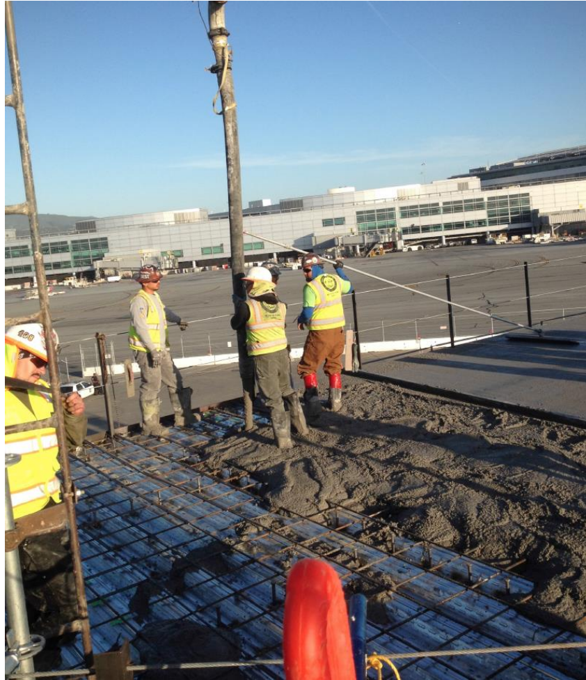
Figure 14.1. Blue Planet Carbon sequestering (carbon negative) aggregate in concrete being poured at San Francisco airport, May 2016
