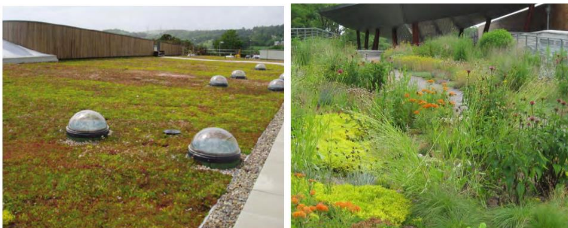
Figure 4.2. Example of extensive green roof (left) and intensive green roof (right) 135
