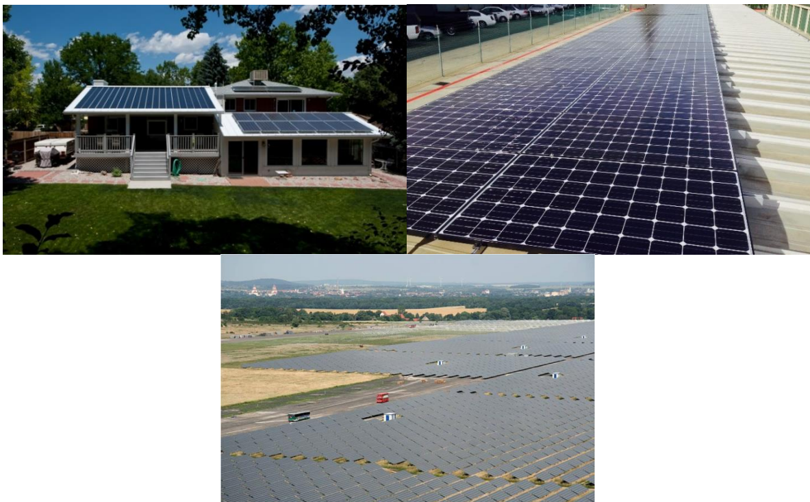
Figure 7.1. Residential PV (top left), 208 commercial PV (top right), 209 and utility-scale PV (bottom) 210
