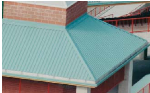
Metal roof - Jerry Uht Stadium, Erie, PA
