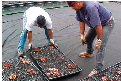
Installation of modular system
