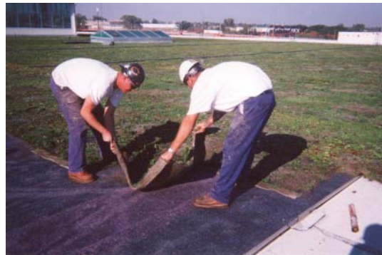
Green roof installation of mats
