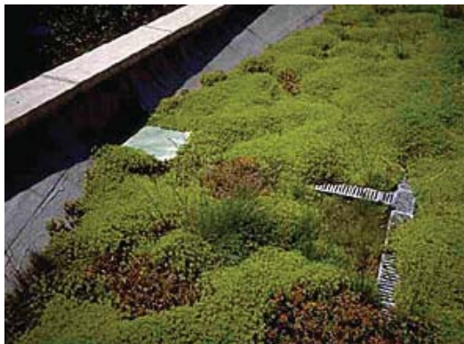
Roof edge, showing drainage elements
