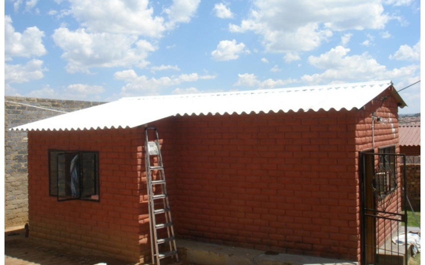
House 4: Cool roof coating and no ceiling
