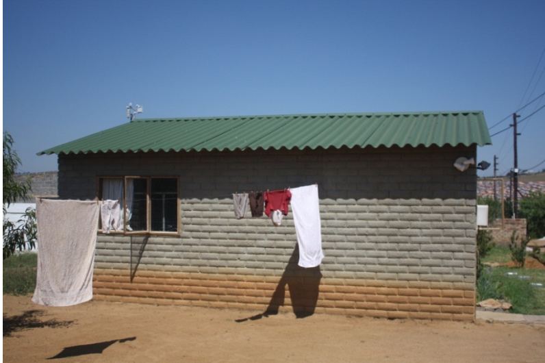
House 3: Newly painted conventional roof coating and no ceiling
