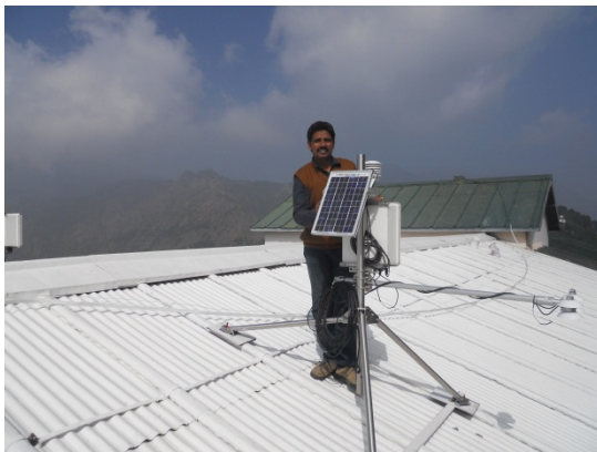
Data monitoring on white roof
