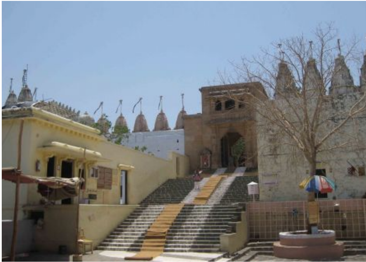
Reflective paint on Pathways, Palitana Temple Complex, Gujarat
