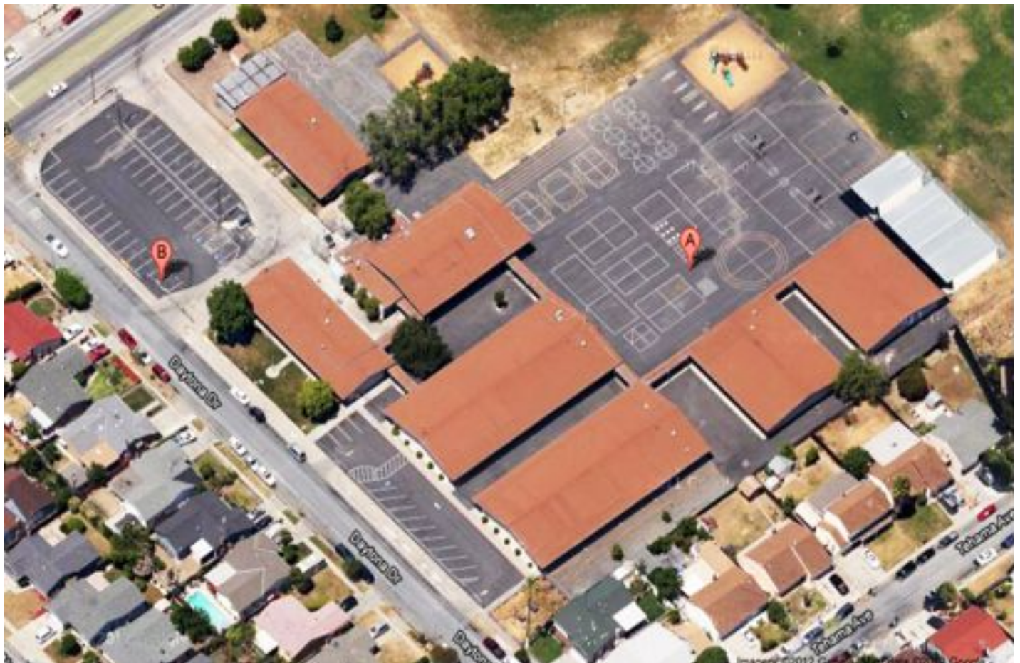
ASPHALT IS HOT - BETWEEN BUILDINGS AND PLAY YARD
