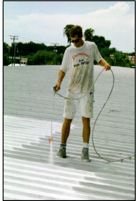
Figure 13. Phase II roof whitening on July 30, 1997.
