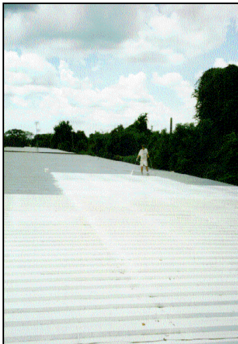
Figure 14. One year old white roof surface (foreground) against freshly coated roof section.
