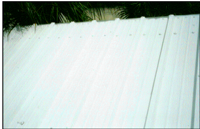
Figure 15. Close-up of one year old white roof section.
