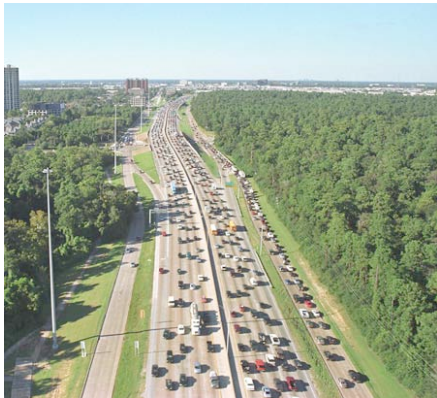
Aerial view of Houston freeway
