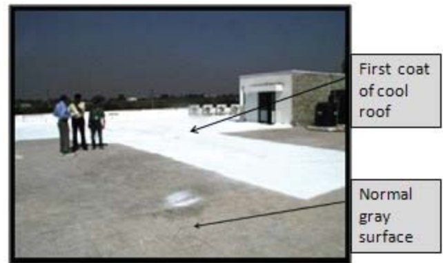
Figure 2. Installation of white coating on the concrete roof
