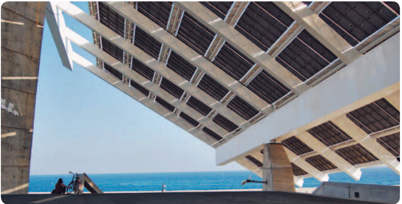
Esplanade and Photovoltaic Power Plant by racEcar_yayas/flickr.com
