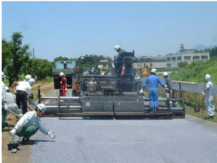
FIGURE 8 View of applying test pavement
