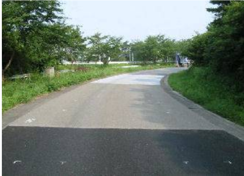
FIGURE 10 View of the completed test pavement
