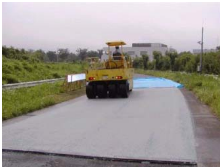
FIGURE 9 View of conducting rolling compaction
