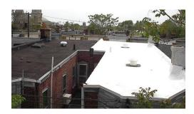
coatings have high reflectance and high emissivity, reflecting up to 92 percent of solar radiation, and shedding heat gain as soon as the sun goes down in the evening.
